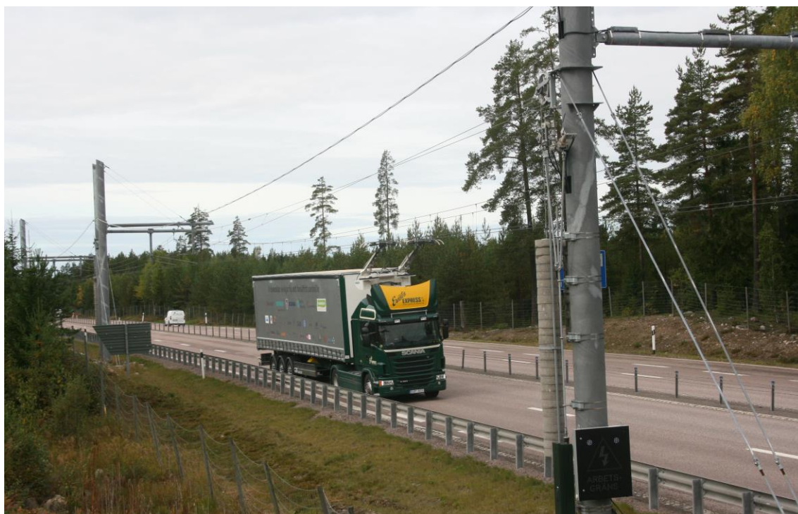
Figure 16. eHighway in Sweden
