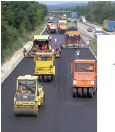
Figure 3: Pavement construction on a motorway
