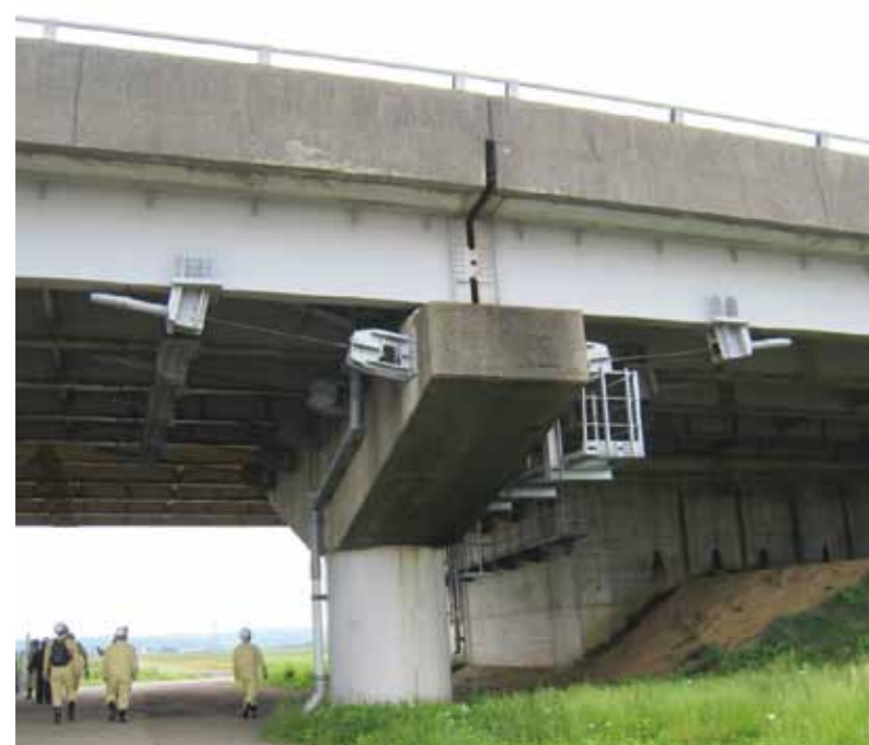
Steel jacking for pier body and unseating prevention devices
