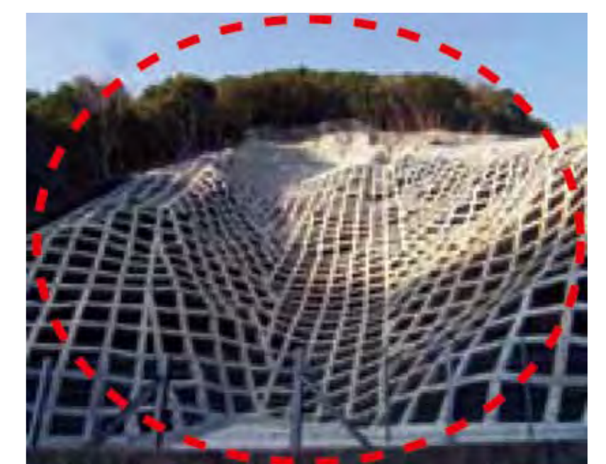
Protective concrete that prevent roadside slope collapsing
