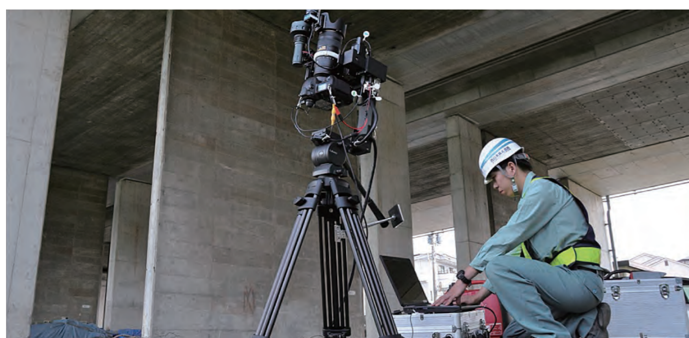
Bridge inspection using Digital Camera System
