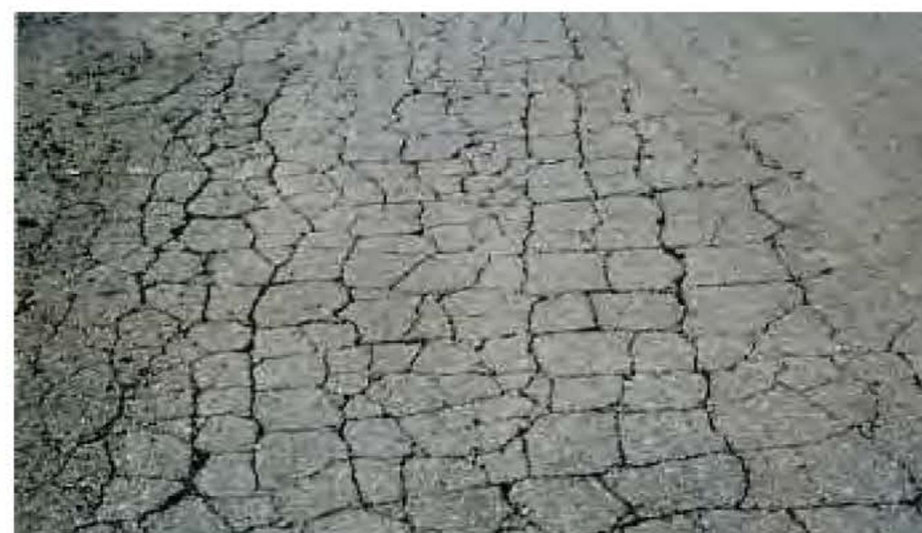
Heavy Goods Vehicle and pavement damage in Laos
