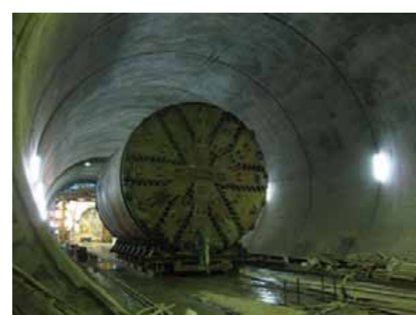
Transfer of the TBM at the pass-through section
