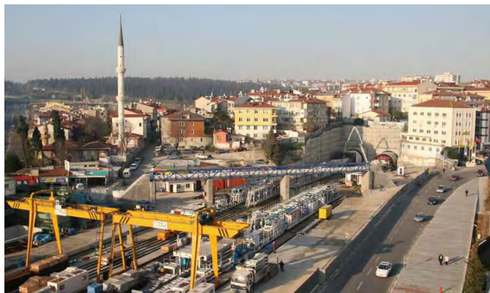
Preparations for the simultaneous start of TBM No. 4 and 5 followed by back-up cars
