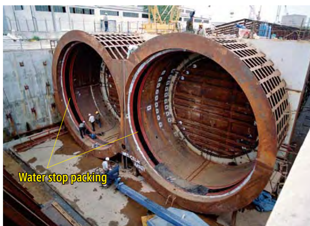
The immersed tube tunnel end is backfilled with artificial foundation to be excavated by TBMs.
