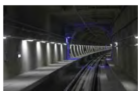
Connection of the immersed and shield tunnels
