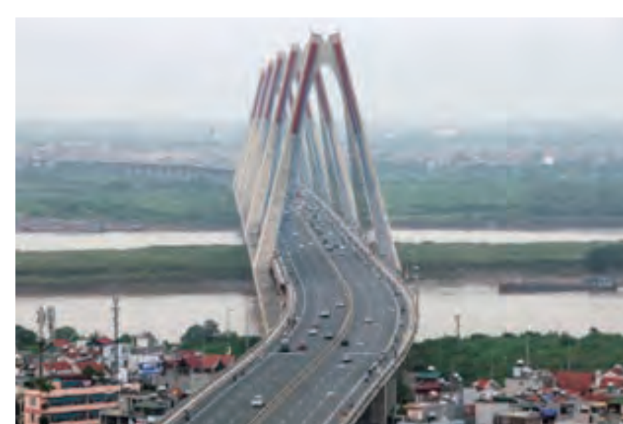
Nhat Tan Bridge (Completed in 2015)
