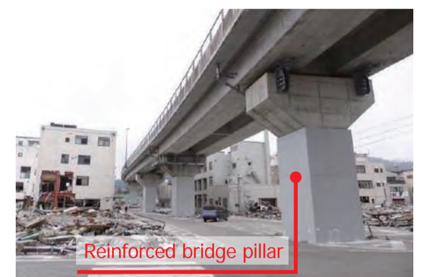
<Bridge with antiseismic reinforcement after the Great East Japan Earthquake in 2011>
