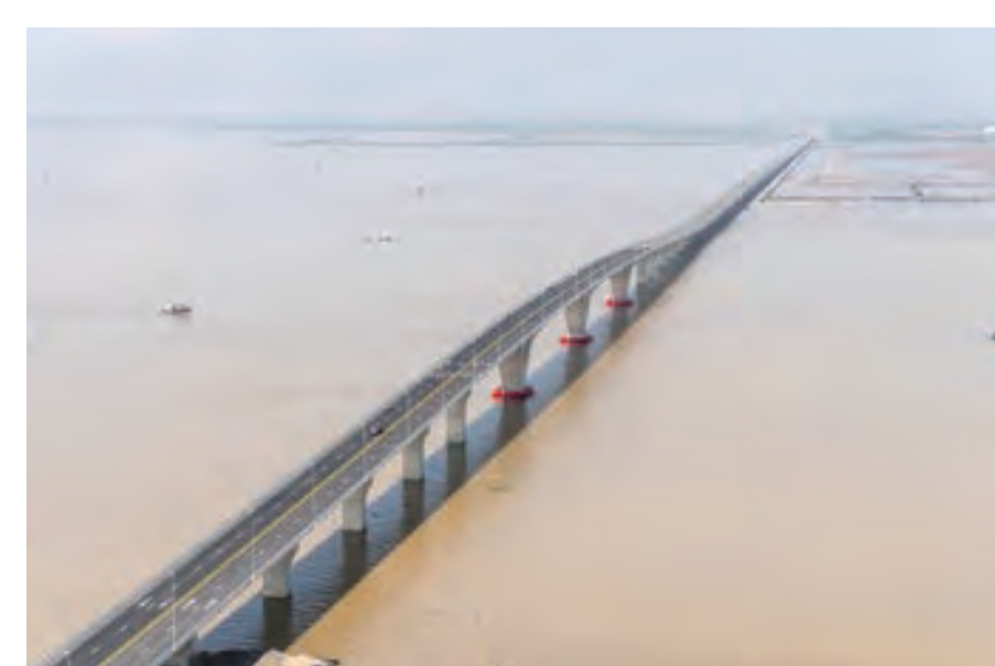
Lucken International Port Access Road (Completed in 2017)
