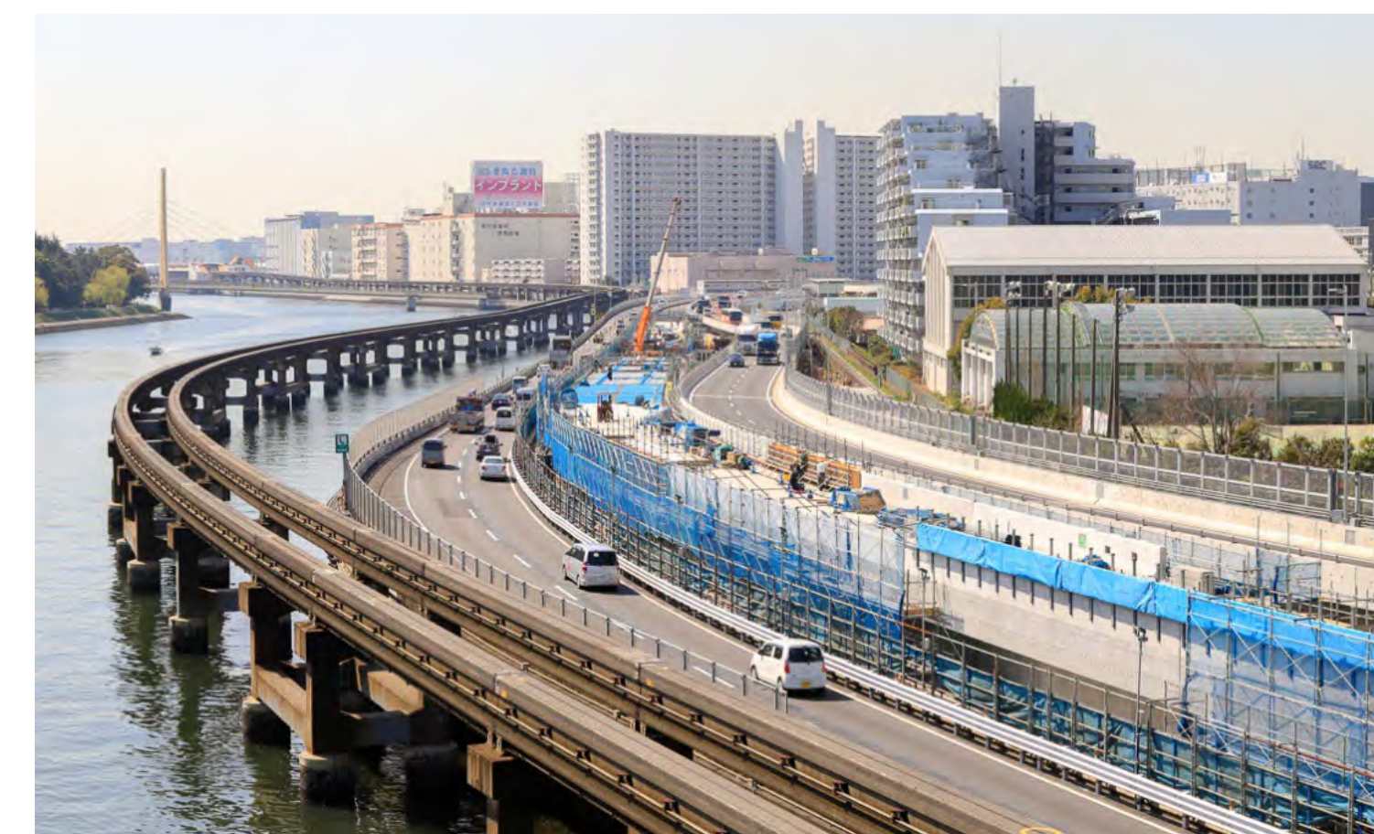
Undergoing Renewal Works (2019)
