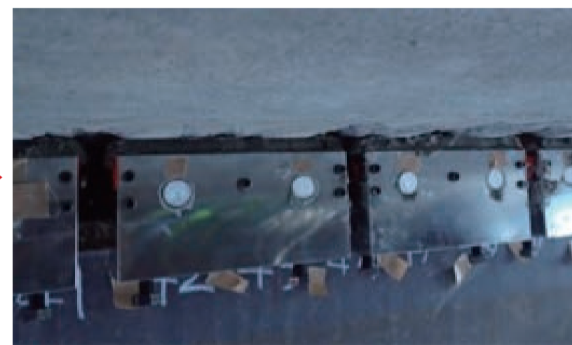
Install temporary reinforcement (flange guard) between the girder and the floor base
