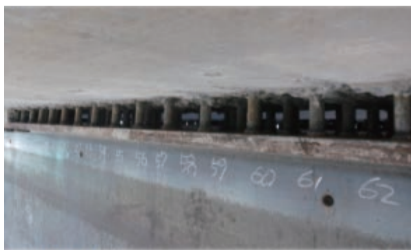
Apply WJ to remove the connecting concrete
