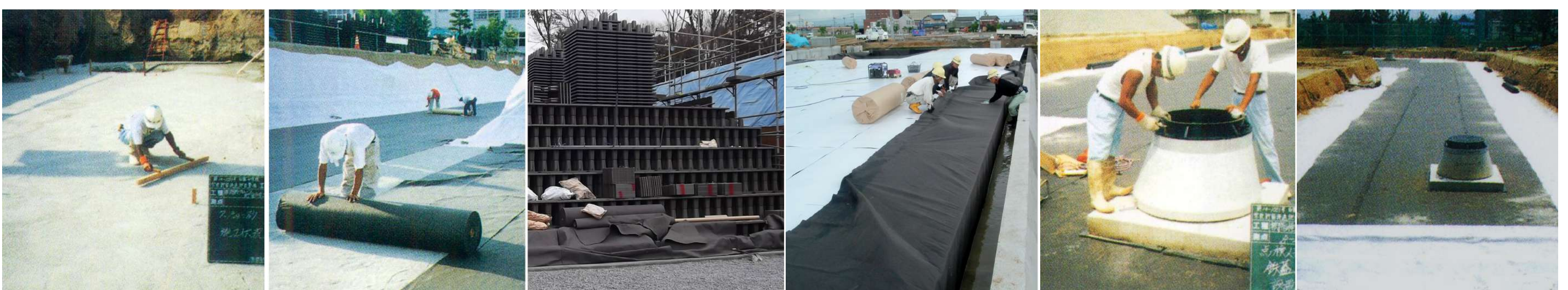
① Foundation work
