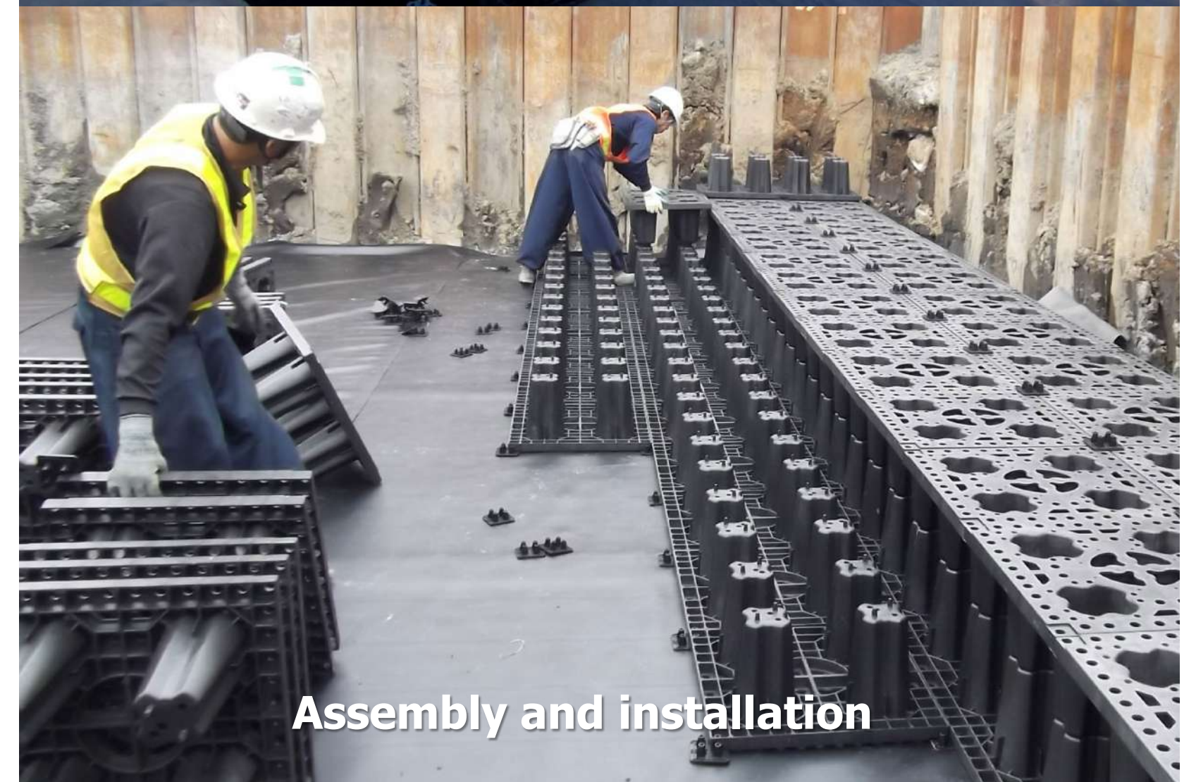
Units being assembled
