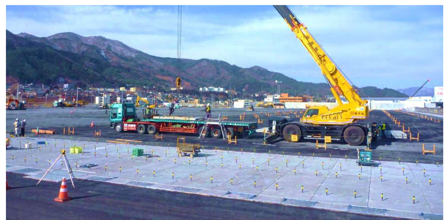
Installation at a seaport pier site
