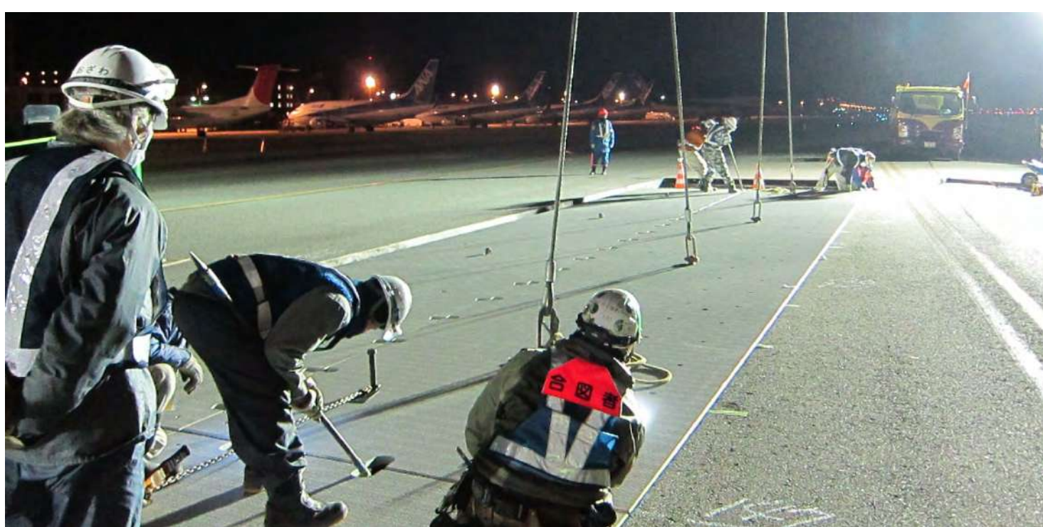
Speedy installation within limited timeframe (airport taxiway)
