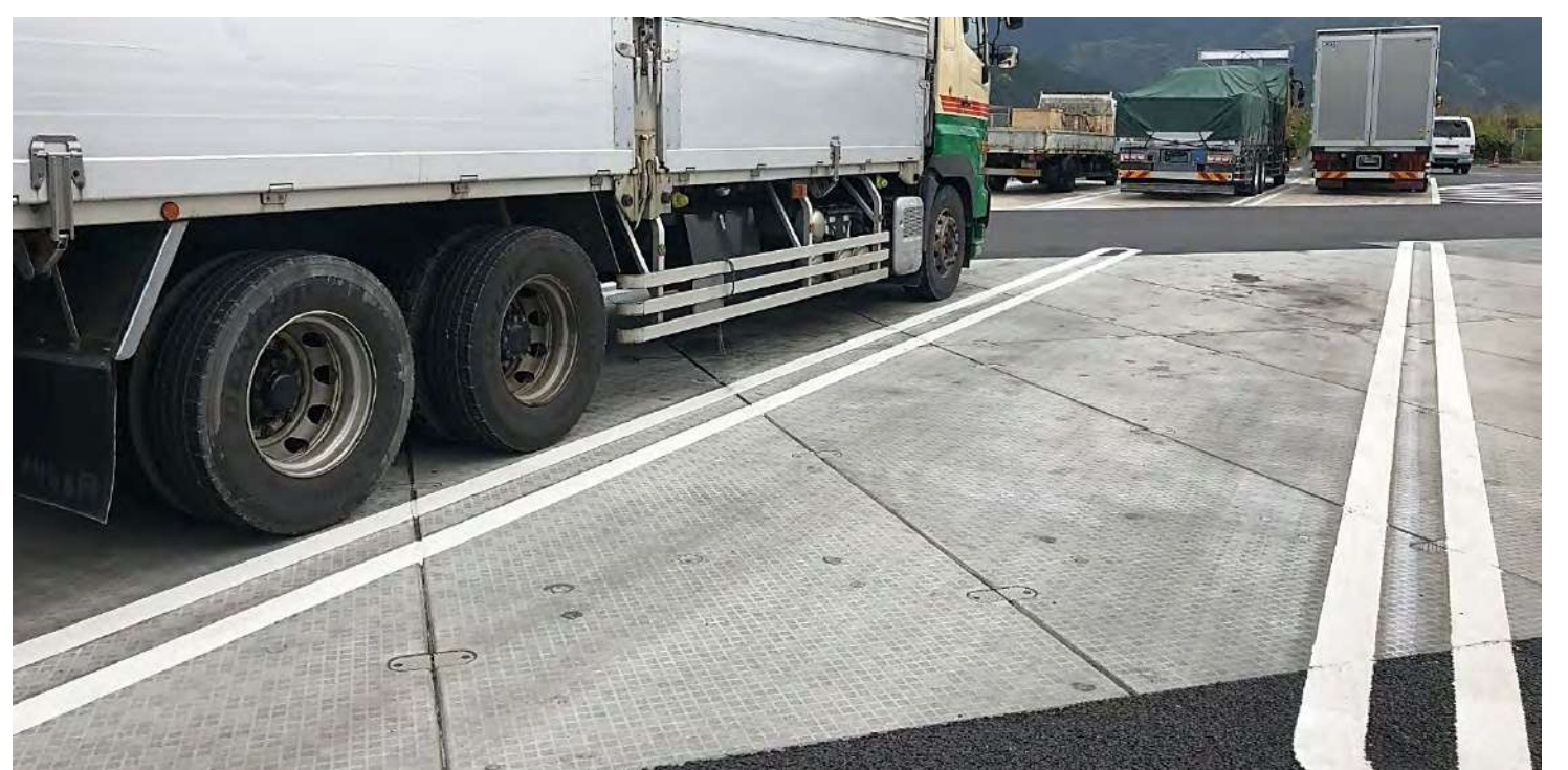
Rutting reduction in large-vehicle parking lots at a highway PA
