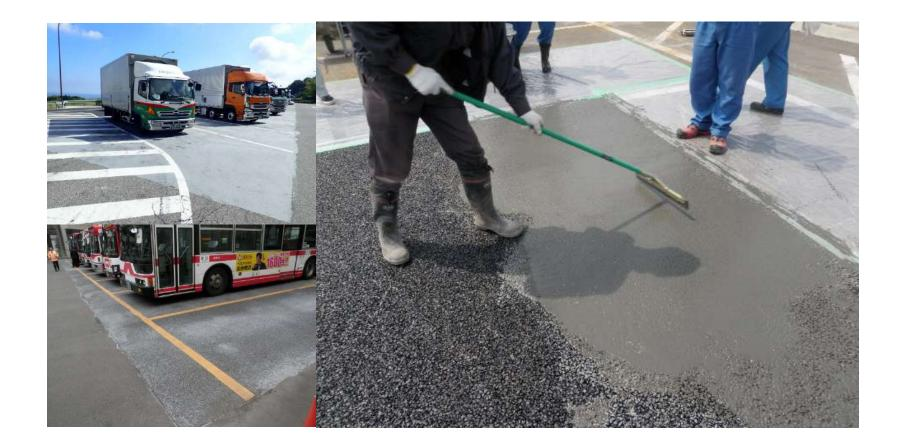
Ultra Pave H is a paving composition that provides good fluidity resistance, oil resistance and resistance to stationary steering while also offering levels of static load bearing capacity that are equivalent to concrete paving. It is a semiflexible paving composition that combines the durability of concrete paving and the flatness and deflection compliance of asphalt paving.
