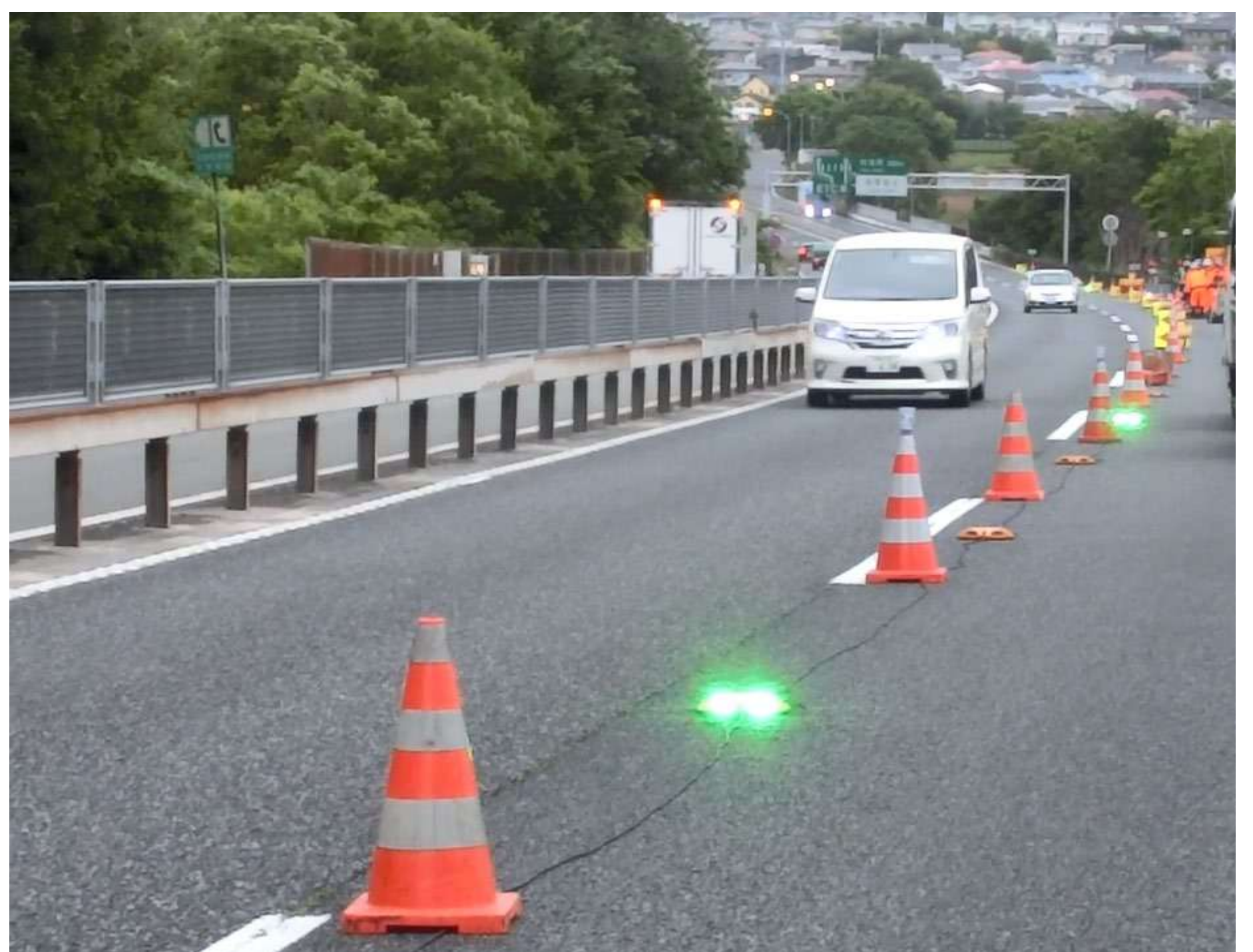
Lane restriction during roadwork
