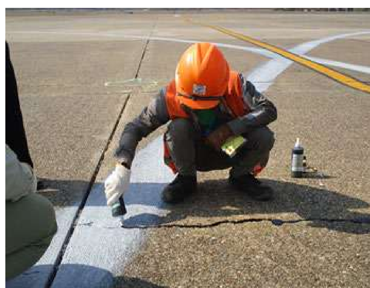
Applying the filler
