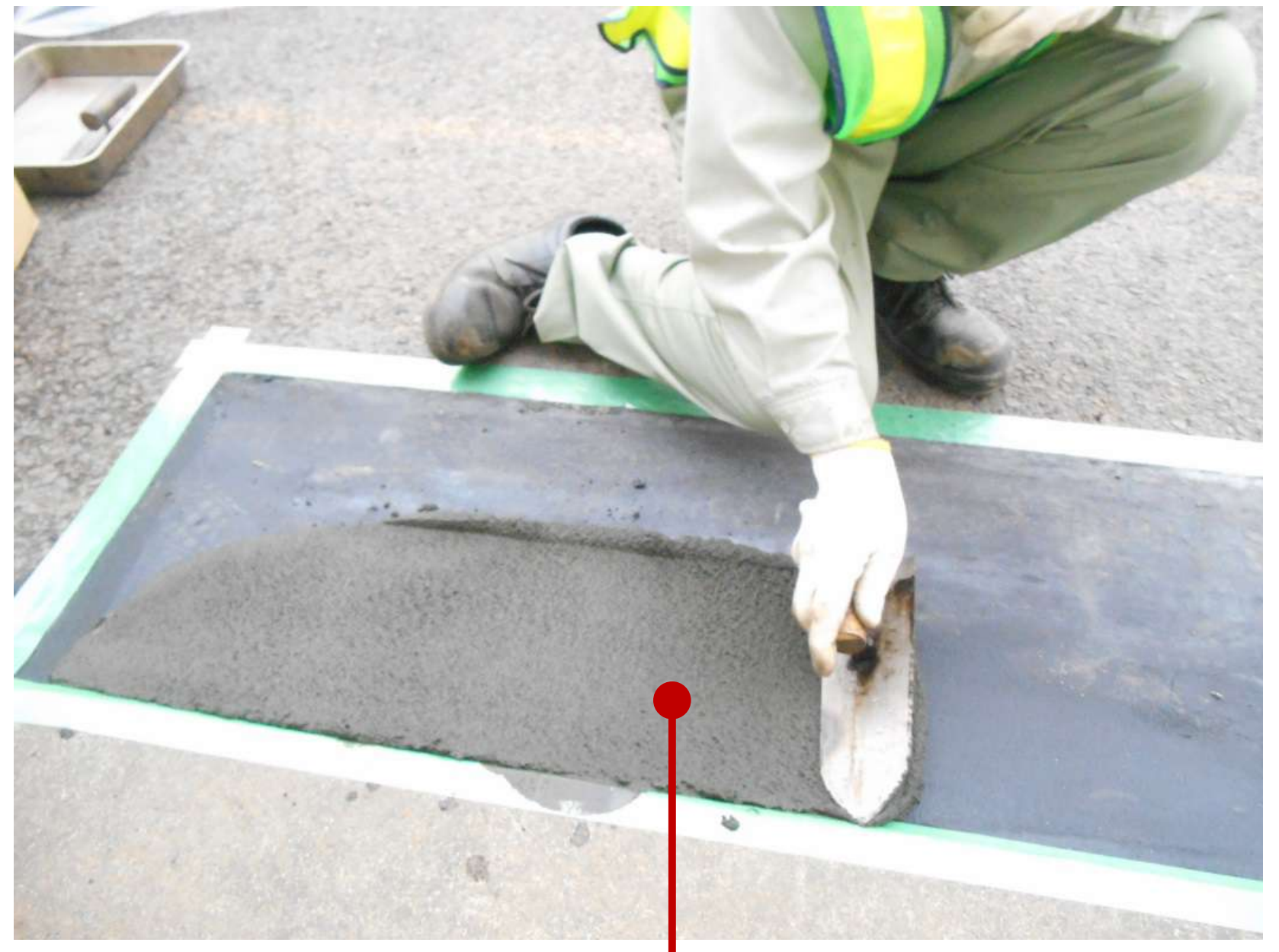
Bumps can be easily plastered over with a trowel.
