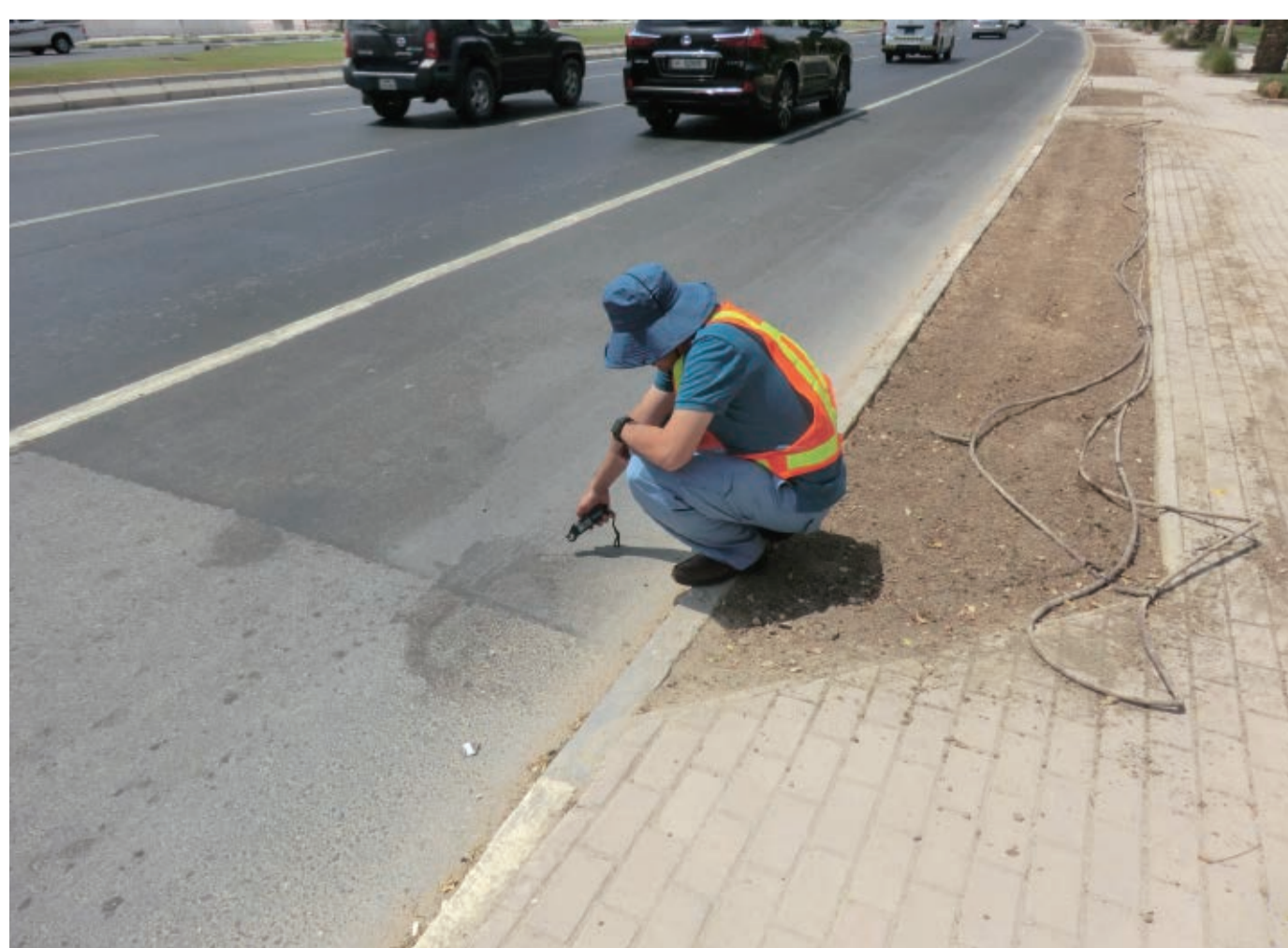
Road surface temperature measurement survey
