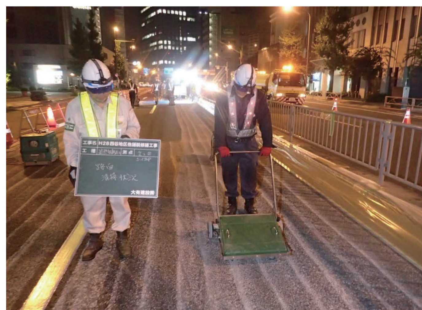
Applying a heat-blocking coating (in Japan)
