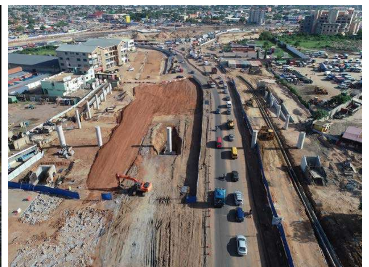
Pedestrian Bridge construction
