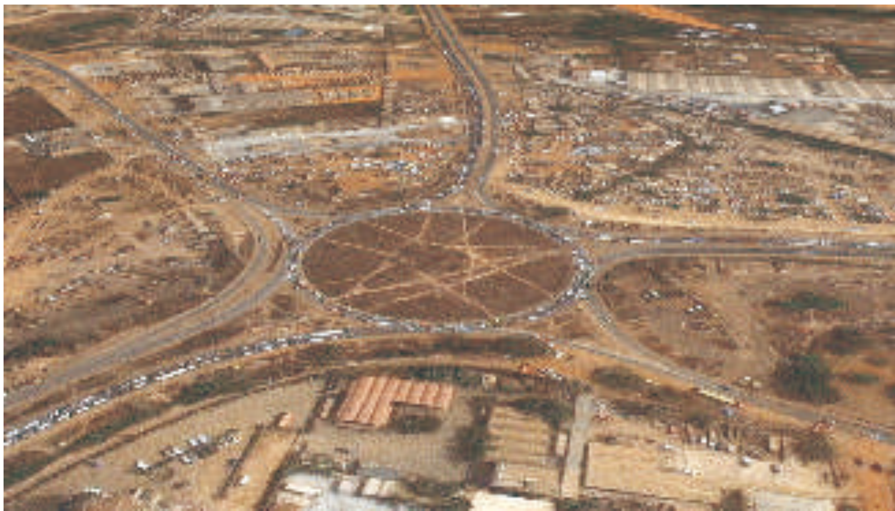
Before work start
