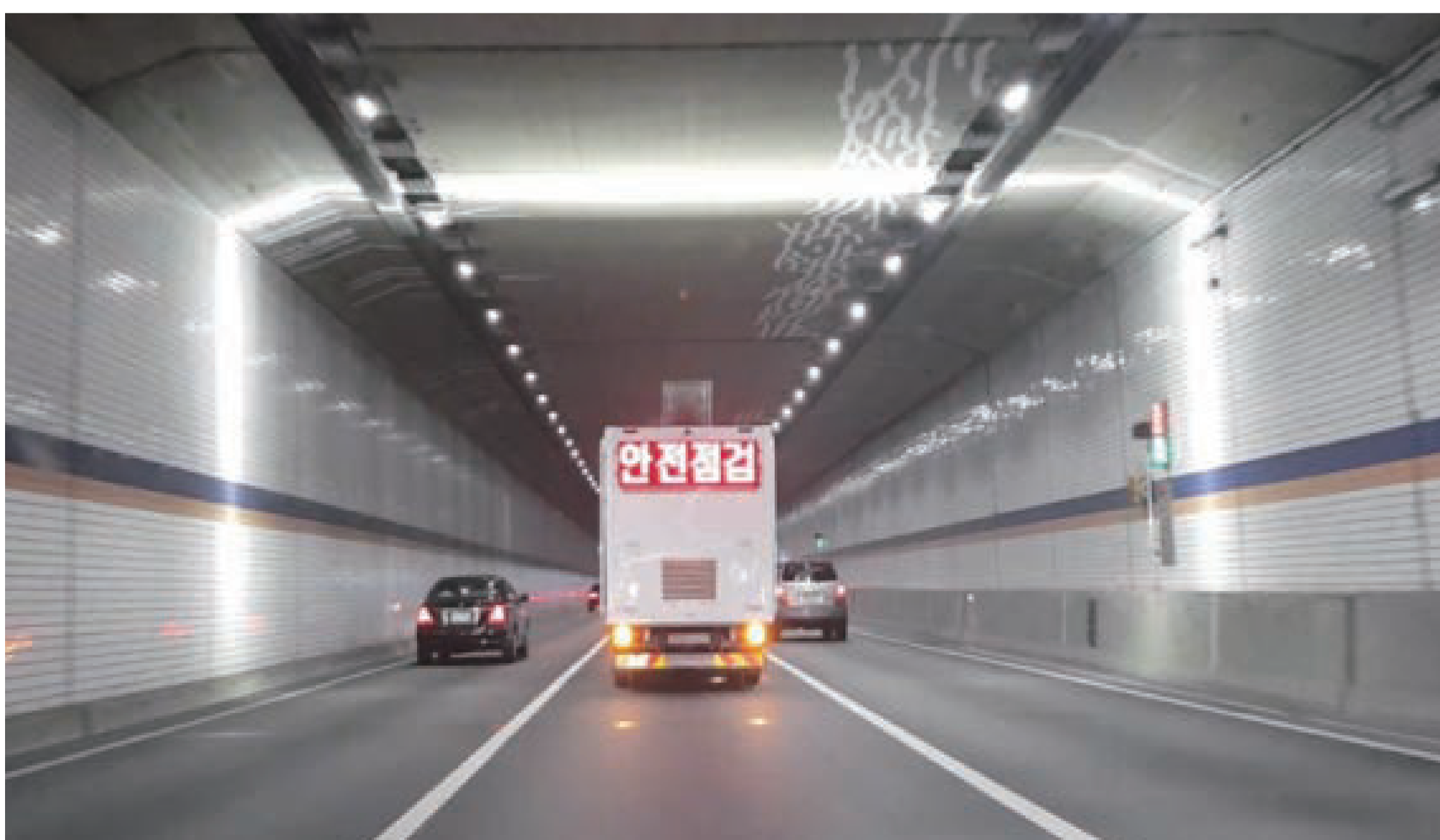
High Speed Scanning Vehicle scan tunnel up to 100km/h.
