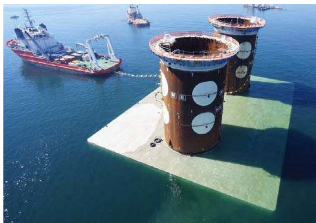
Steel Shaft for tower foundation
