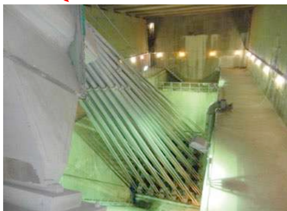
Spray room in anchorage
