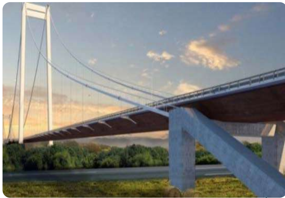
Ongoing Braila Bridge (2018~, Romania)
