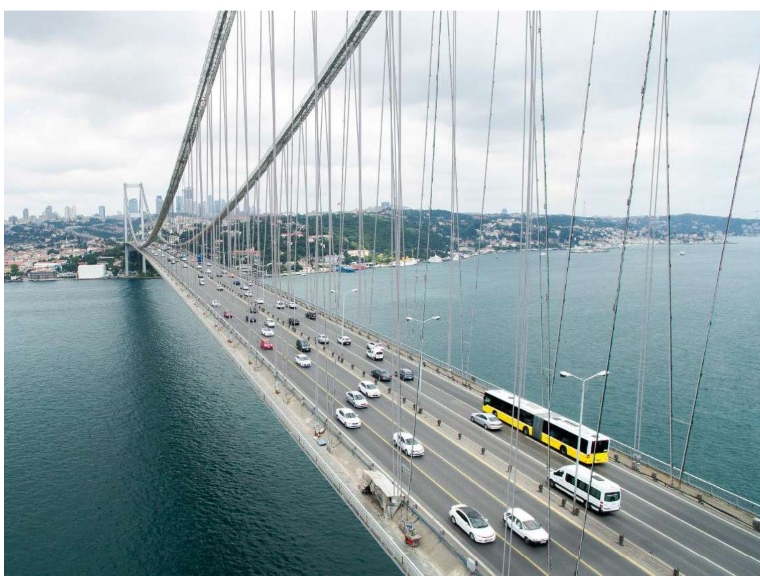
Inclined cable and gusset plate (Before the replacement)
