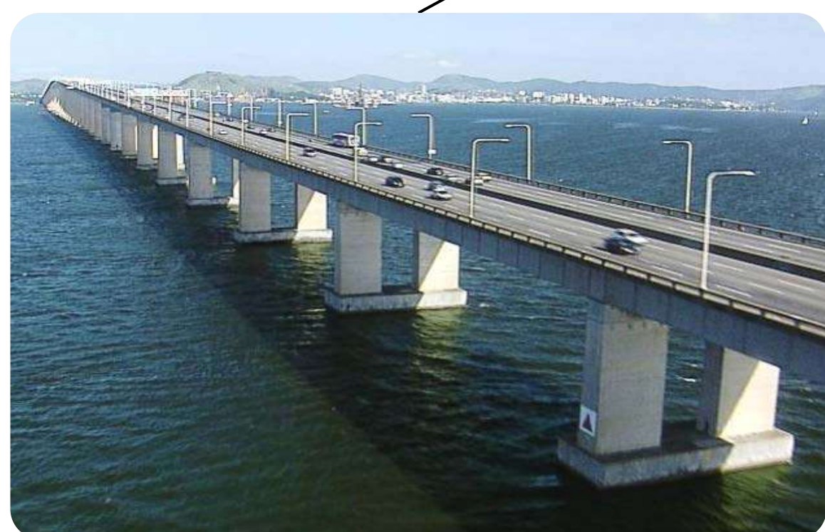
Ongoing Mumbai Trans Harbour Link Project (2017~, India)
