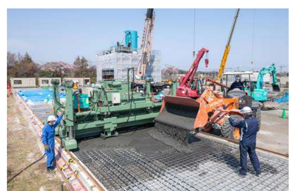
Construction by machine
