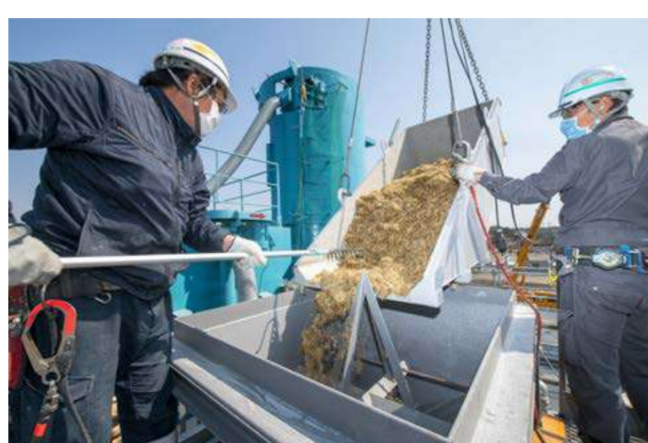
Mixing steel fiber into the concrete mix
